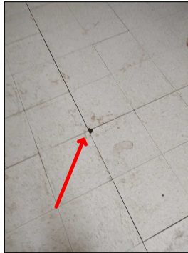
Damaged floor
