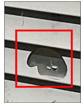
Damaged siding
