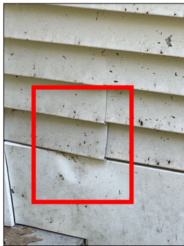
Damaged siding
