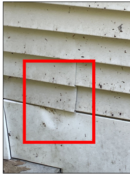
Damaged siding
