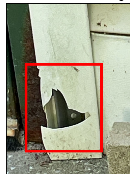
Damaged siding
