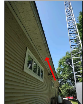
Soffit vents
