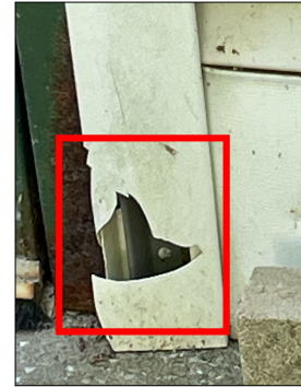
Damaged siding
