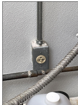
Receptacle that needs to be GFCI protected
