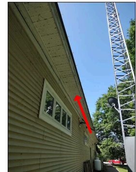
Soffit vents
