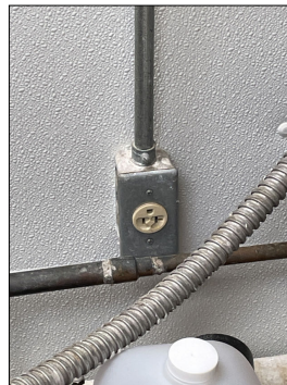
Receptacle that needs to be GFCI protected
